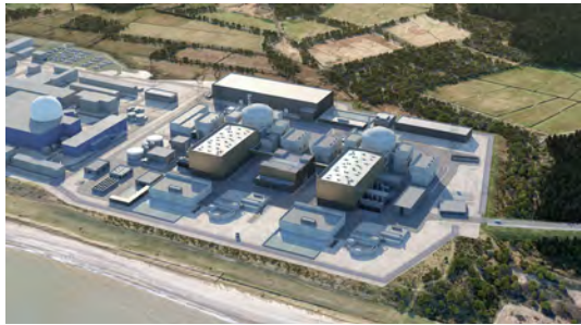
Aerial view of Sizewell C Operational Site
